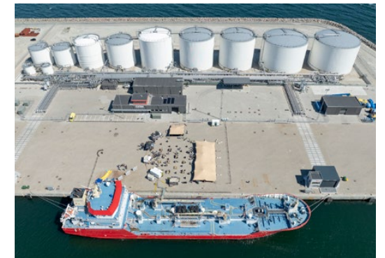
Stena Oil’s new marine fuel terminal in Frederikshavn, Denmark, was inaugurated on May 14, 2024.
